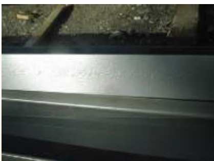
Img. 2.6.1. Smashing through of the scarred surface
