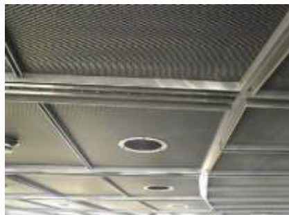
Img. 6.4.2. Cloud formation caused by different film thickness
