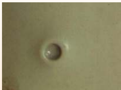
Img. 2.4.5. Bubbles caused by tassels in the galvanized plate
