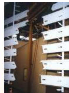
Img. 1.2.3. Create an additional earthing
