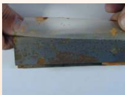
Img. 5.3.5. Infiltration caused by an insufficient pretreatment
