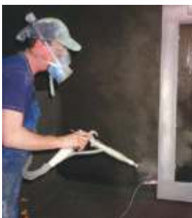
Img. 1.5.1. Additional earthing for hollows
